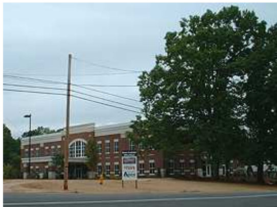
Presbyterian, Building One on north end of property
