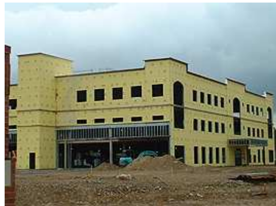
CMC Building under construction
